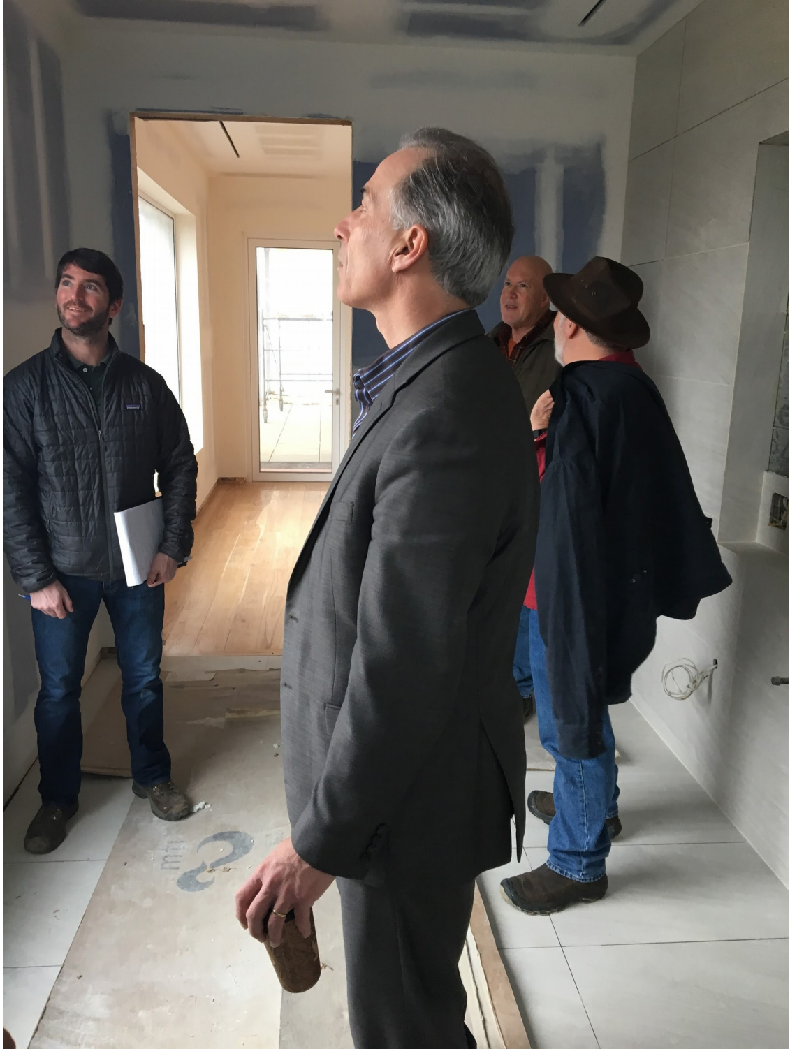
Town of Red Hook Energy Code building site visit, site 2, Town Supervisor Robert McKeon center (Laurie Husted)
