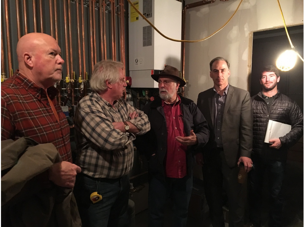
Town of Red Hook Energy Code building site visit, site 2, Town Supervisor Robert McKeon 2nd from right (Laurie Husted)
