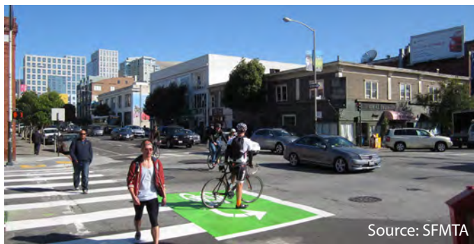
Two-stage turn queue boxes provide a holding area for bicyclists to queue, allowing them to cross an intersection in two stages. This crossing pattern is more comfortable, especially for less experienced bicyclists
