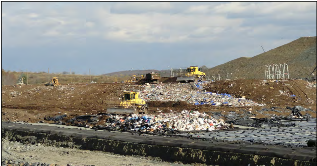
Photo 5: 2017 Landfill Working Face – Section VI Cell 3.
