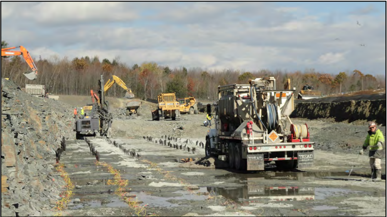
Photo 6: Landfill Section IV- Cell 4 Shale Blasting
