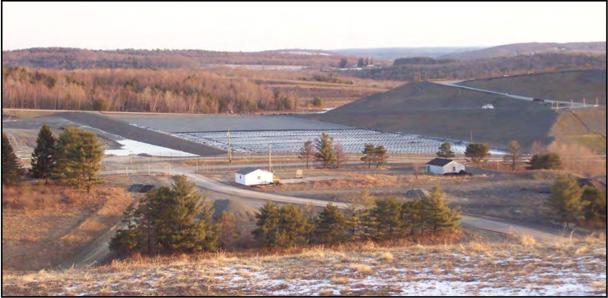
Photo 1: Landfill Section IV – Cell 3
