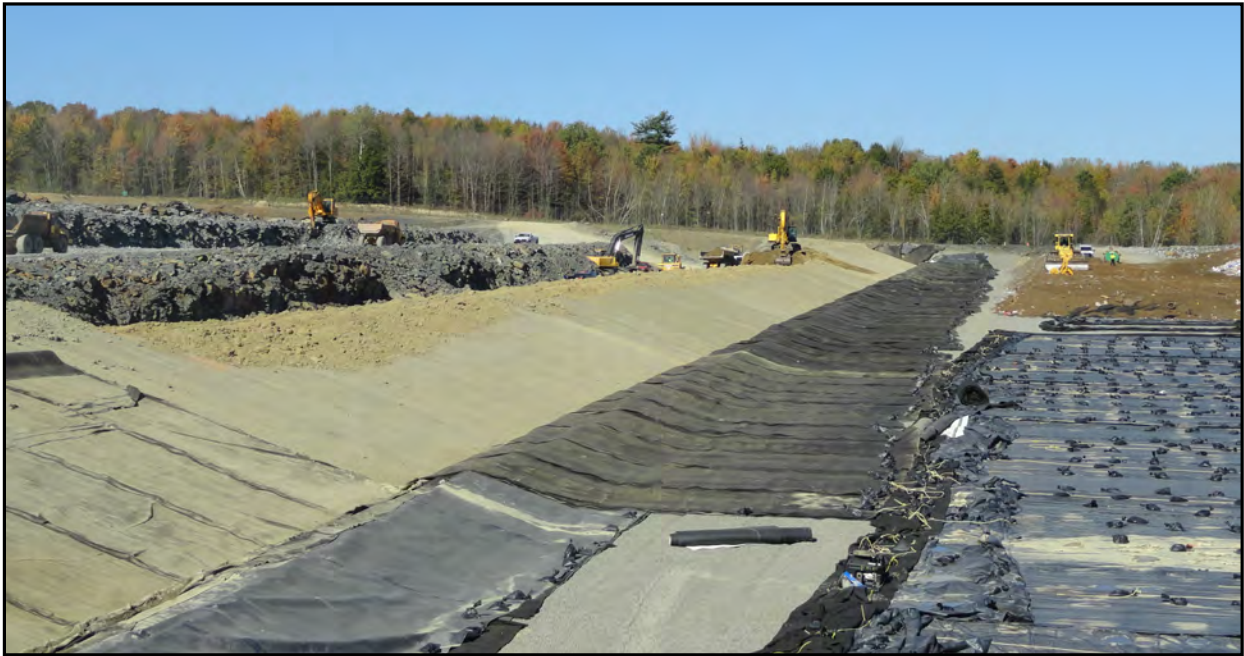
Photo 7: Cell 3-4 Berm Reconstruction
