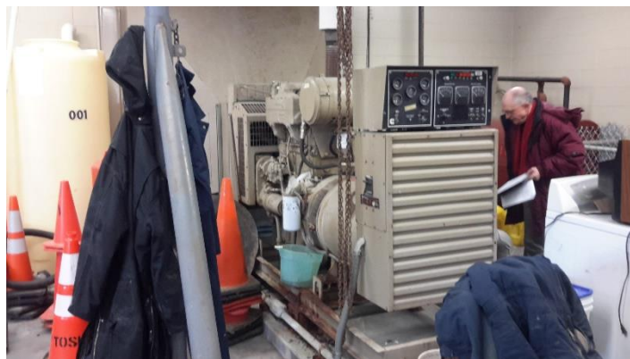
Figure 13: Standby generator in the control room
