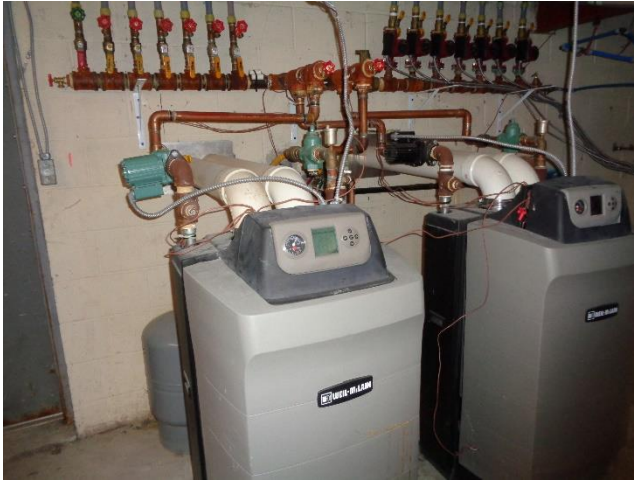
Figure 19: Weil-McLain 299 MBH boilers (left) and Bosch 151.6 MBH boiler (right)
