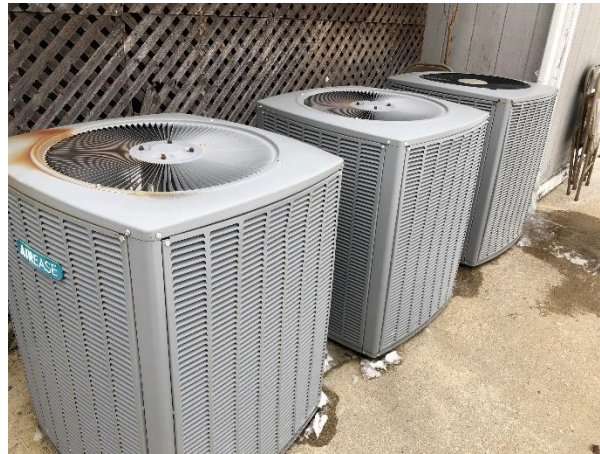
Figure 29: Cooling condensing units
