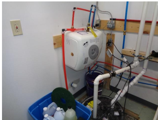
Figure 23: Instantaneous water heater for the Helsmortel Wing
