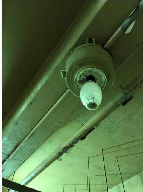
Figure 5: Metal halide light fixture in the pump room
