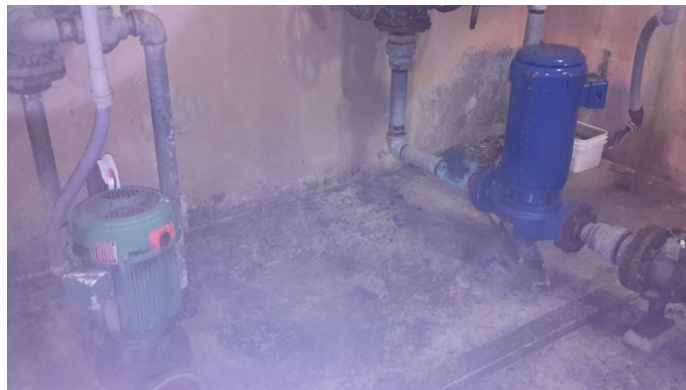
Figure 11: Booster pumps in the pump room
