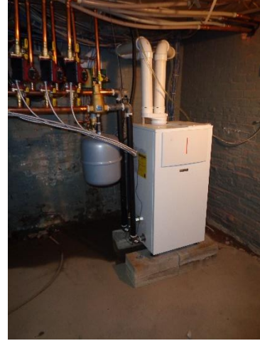
Figure 19: Weil-McLain 299 MBH boilers (left) and Bosch 151.6 MBH boiler (right)
