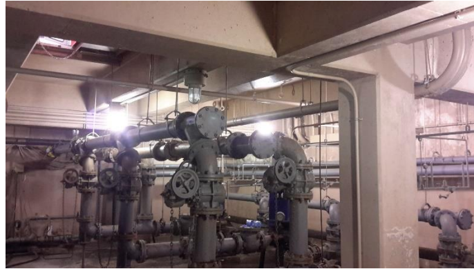
Figure 10: Recirculation pumps in the pump room
