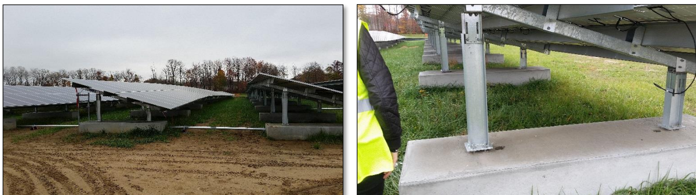
Figure 1. - Fixed Axis Solar PV Array on a ballasted concrete foundation
