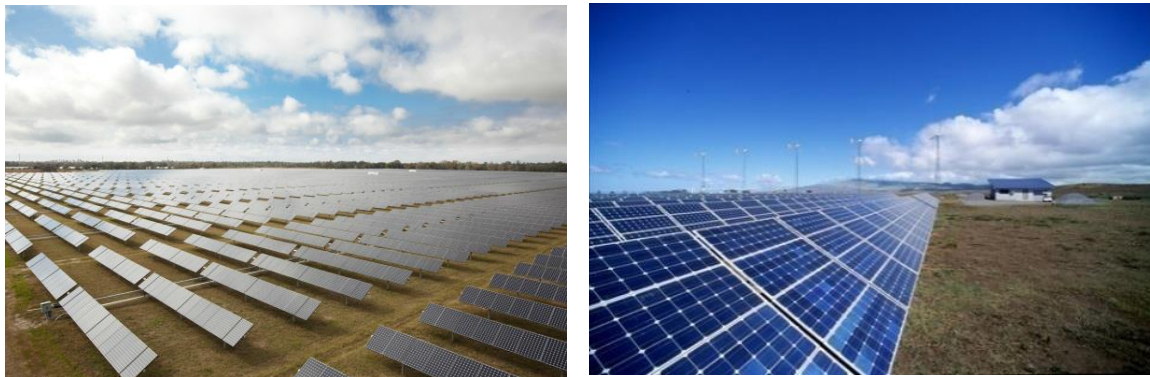
Figure 8. Mono- and multi-crystalline solar panels. Photos by (left) SunPower Corporation, NREL 23816 and (right) SunPower, NREL 13823
