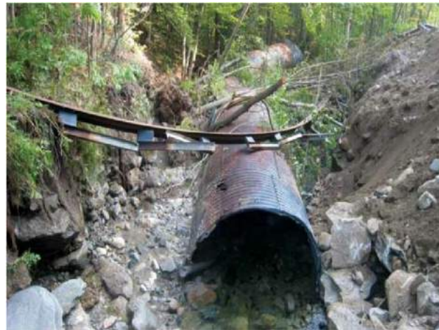
Road failure at a 3-m culvert placed within a 6-m bankfull width stream, GMNF
