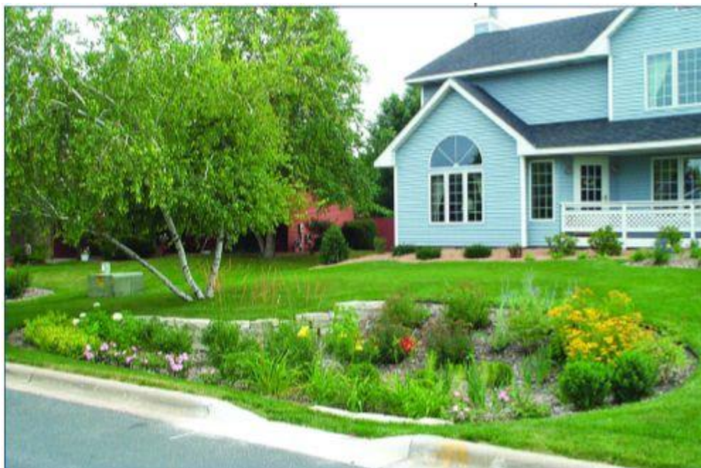
Figure 16. A rain garden strategically placed at the end of a yard, in order to capture street and lawn runoff.
