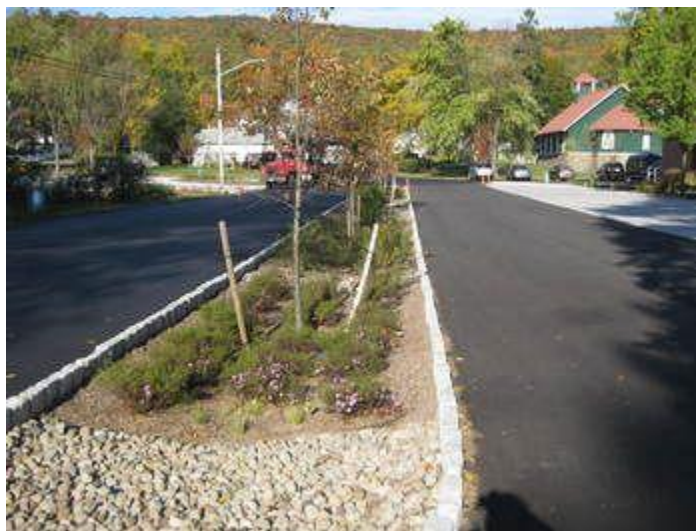
Figure 15. A Vegetated swale in the median of a roadway in the Village of Greenwood Lake in Orange County. (NYSDEC, 2018a)
