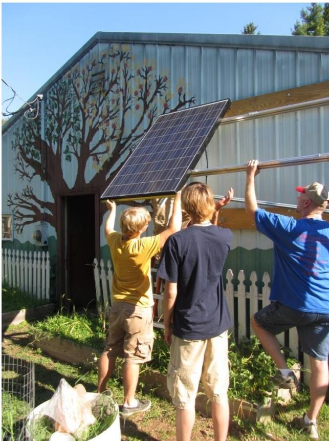
either end so before anything was screwed in, 20 bolts were slipped into the top rail, and 10 on the bottom rail. The top rail requires more bolts because it supports each solar panel in two places, and it also houses the micro inverters.
