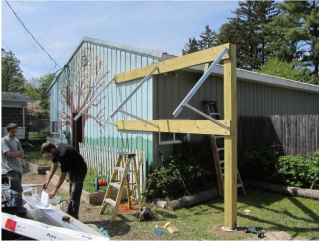
Installing the Solar Mount was as simple as following the instructions included with the unit. First the 6 wall brackets were strategically placed precisely where they were supposed to go. Next the
