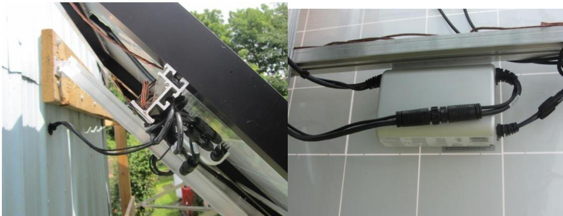
Once the panels were fixed, we began installing the micro inverters. The inverters were tricky to get into place. The ground screw would rest in the channel of the rail, so the entire inverter had to be lifted up and placed into the rail, it then had to be held there while bolted into place. This process was repeated for the five micro inverters.
