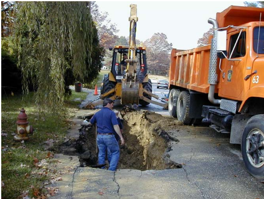
A water project in Cortlandt
