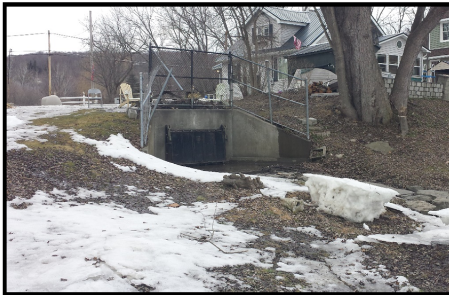
Looking West at the Stormwater Channel Outfall
