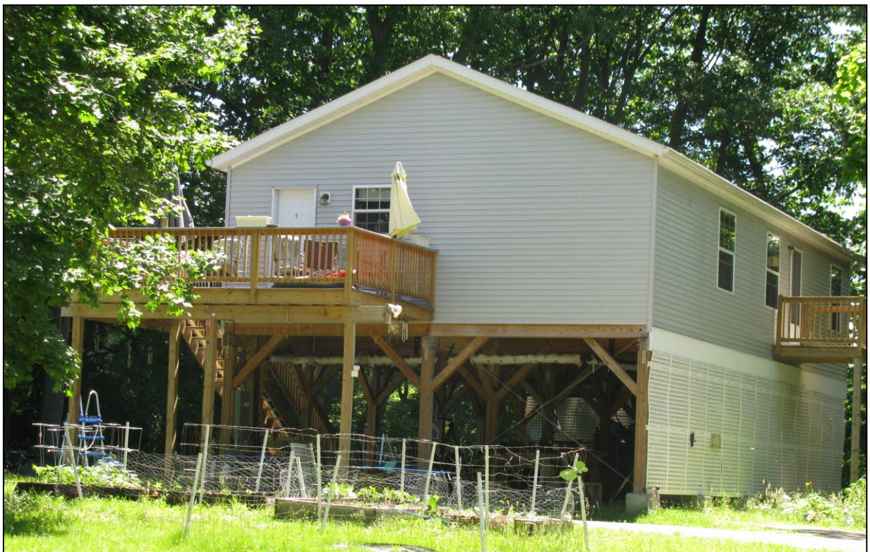
Elevated home in the Town of Conklin (2016)
