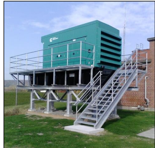
Right: JC Water Treatment Plant with new back-up generator elevated above flood levels (2013)
