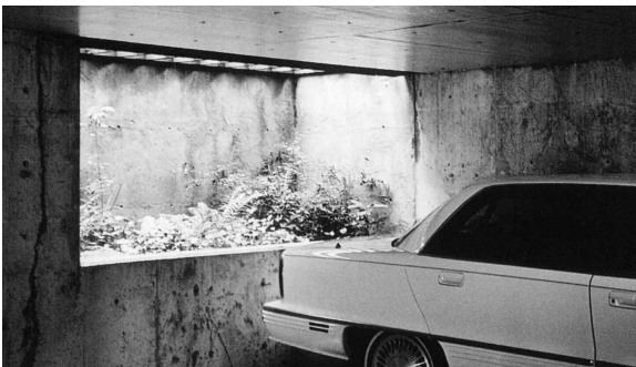
Above: A parking deck recessed into the hill behind Village Hall also provides the opportunity to restore two blocks of the Old Croton Aqueduct Trail, provide a space suitable for green market and Historical Society events, and employ landscaping to hide the lot from view.
