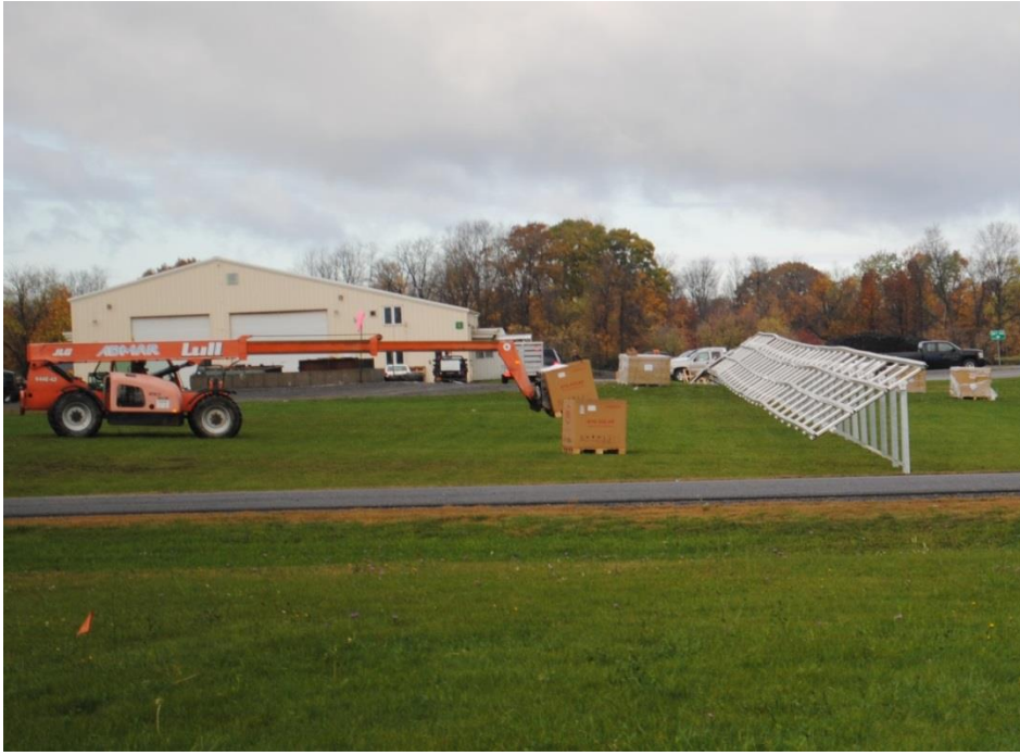
The panels arrive.
