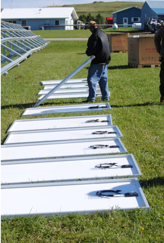
Crew members are getting ready to set up the panels.
