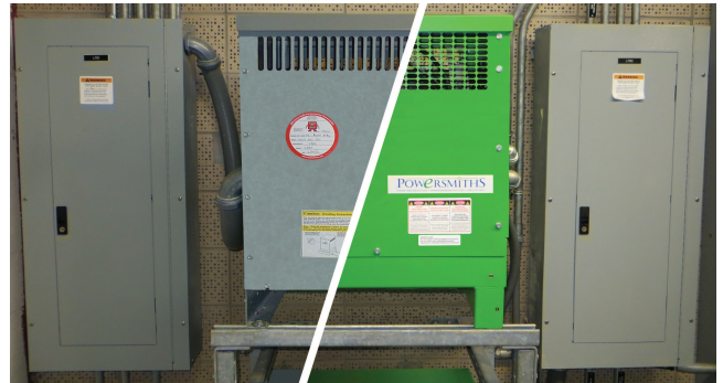
45 kVA E-Saver 2016-R shown replacing an existing 45 kVA transformer. The E-Saver 2016-R was configured to fit within existing physical and electrical constraints to embed significant energy savings, reduce installation costs, and support a smooth and effective retrofit
