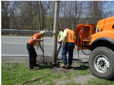
Catch Basin Cleaning
