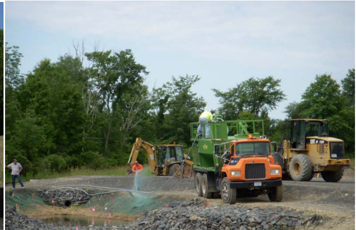
Hydroseeding Stormwater Pond Embankment
