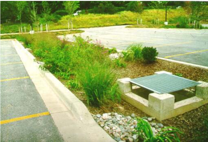
Bioretention Strip
