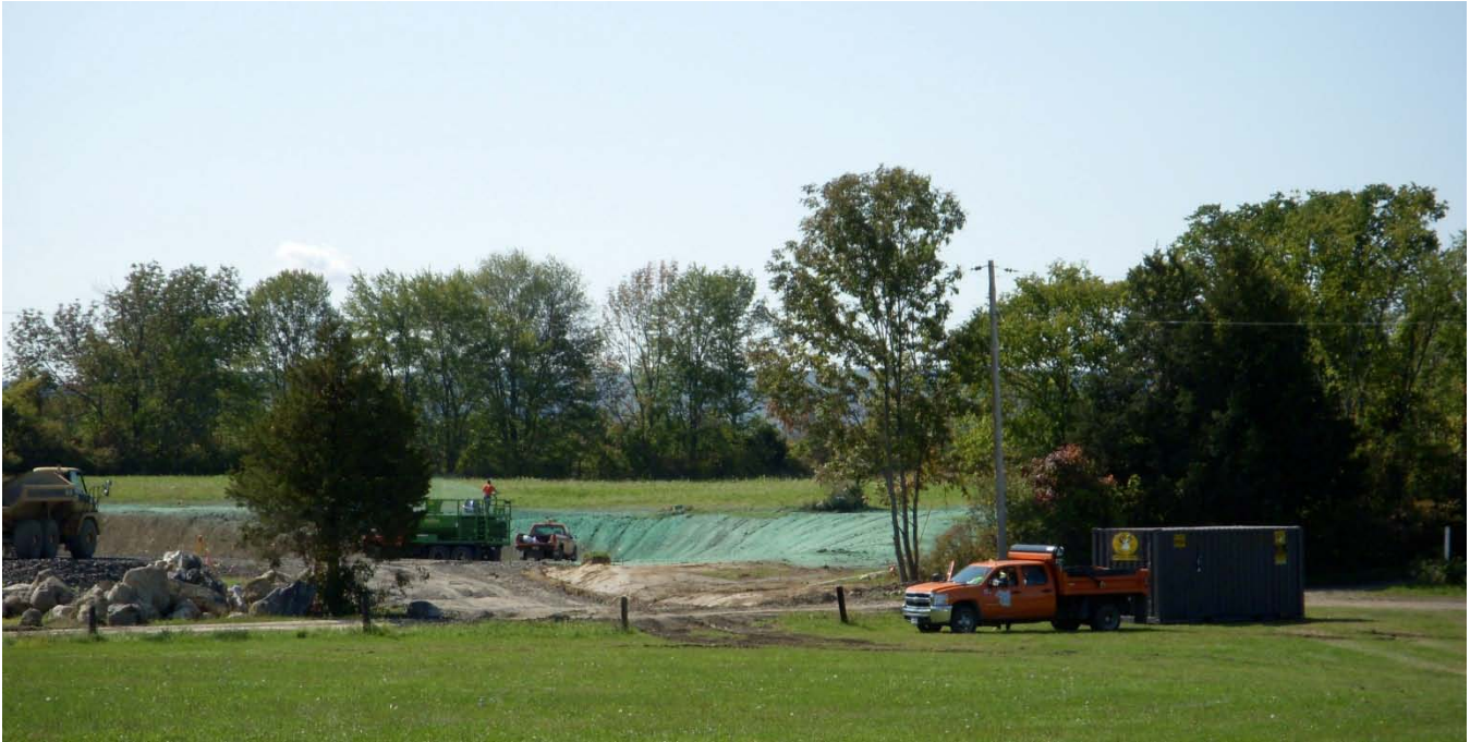
Hydroseeded Slope Stabilization
