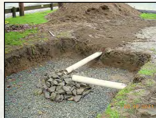
Drain pipes coming from roof, entering garden area
