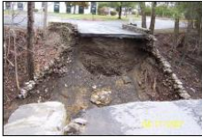
New Rulitz, April 2007: Washout of the sole means of access and egress to the Mountain View Nursing and Rehabilitation Center.
