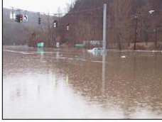
Town of Ulster, April 2005: Flooding of State Route 28.
