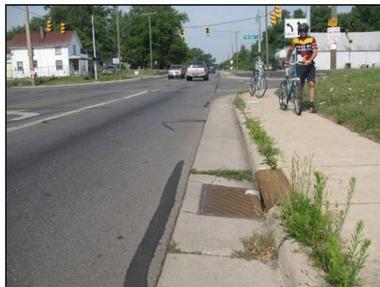
*Roadway resurfacing should ensure that the transitions between the asphalt sections, drainage inlets and other roadway elements are safe and will be maintained for all users.*
