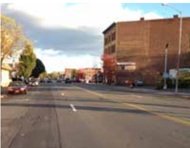
Broadway, west of the rail-road, is 60 feet wide from curb to curb and has existing sidewalks on both sides
