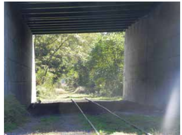
One of the tunnels along the Uptown Corridor
