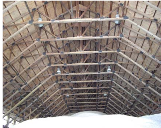
Salt Storage Facility at Boiceville
