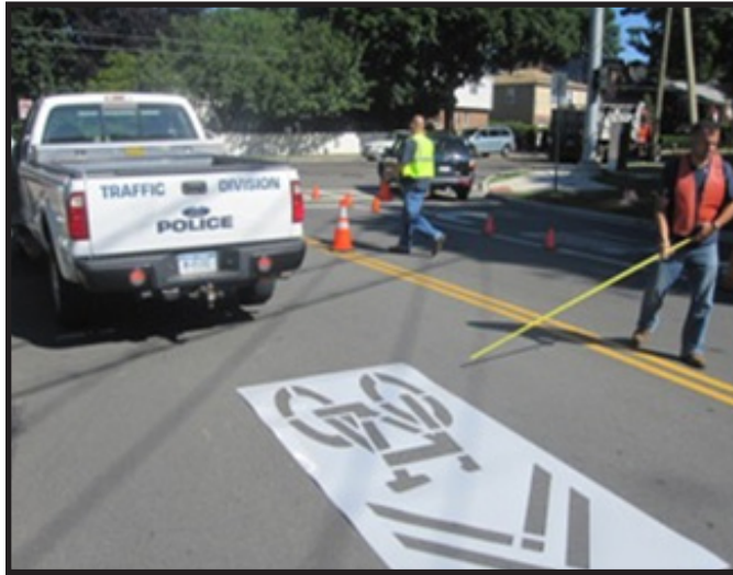
Painting Sharrows on a road in Eastchester, NY cost approximately $200 for a stencil and paint. 49
